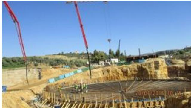
Base Slab Concrete Placement Secondary Clarifier
